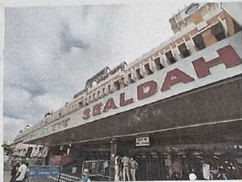
Fig 4 | Outside Sealdah Railway station
